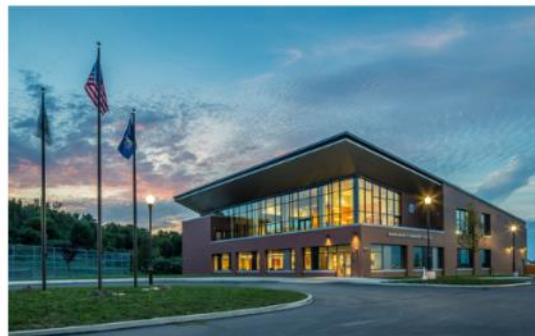
North Fayette Township Community Center
